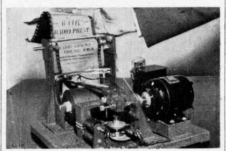
An example of WOR's first facsimile broadcast. A key station of the Mutual network, WOR is located in New Jersey, has 50,000 watts power
